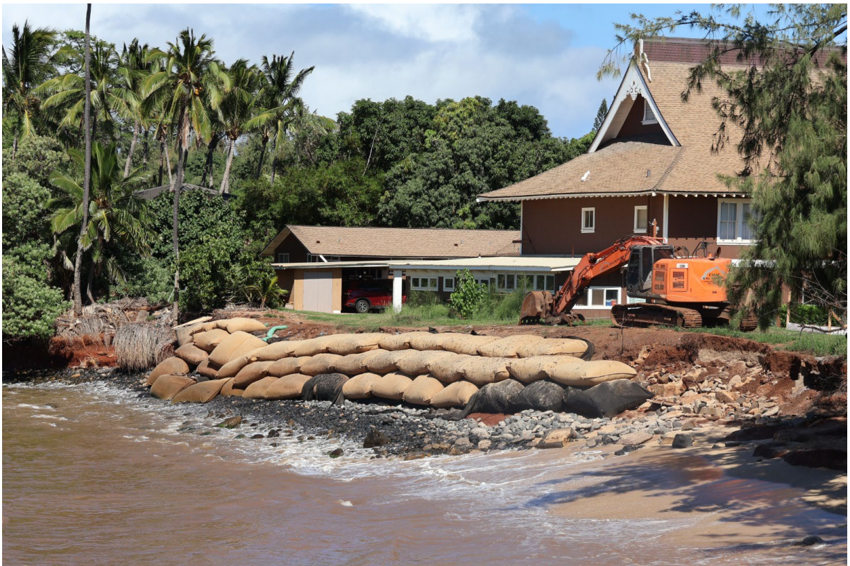
Figure 1 Sandbags used for temporary erosion control at Mantokuji Bay
