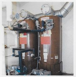
Microprocessor control units, installed on boilers and hot-water heaters, assimilate operating data and automatically determine how long to keep the unit in its "off" cycle, reprogramming the equipment to perform more efficiently.
