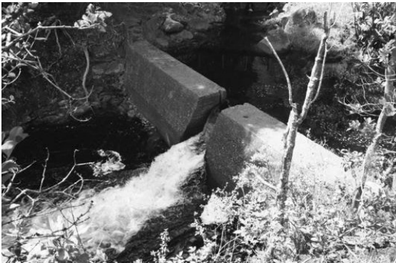
C) Diversion dam at Kauaikinanā Stream.
