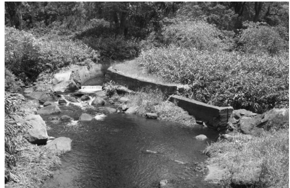
D) Diversion dam at Kōke'e Stream.
