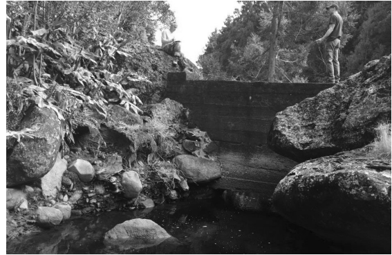
B) Diversion at Kawaikōi Stream.
