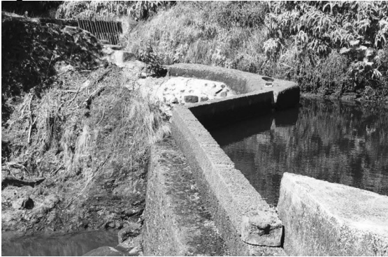
A) Diversion dam at Waiakoali Stream.
