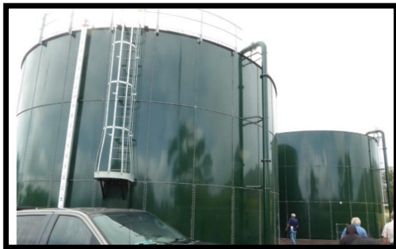
➤ New 228k-gallon steel tanks
