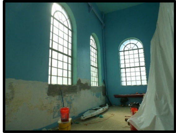
▲ Repainting at the Kalihi Pump Station
