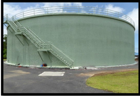
▲ New 2.0 MG tank
