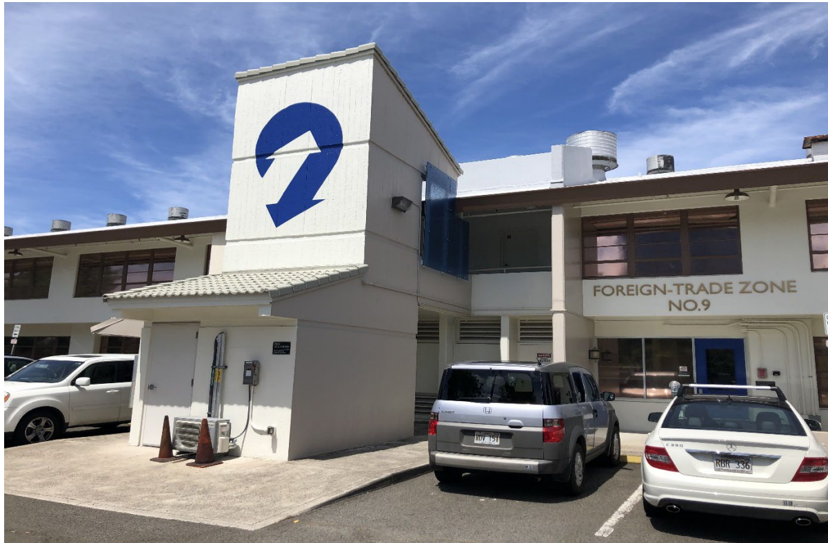
Pier 2 Facility at Foreign Trade Zone 9
