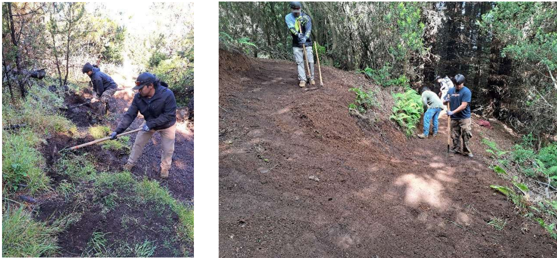
Figure 2. SCA members performing trail maintenance.
