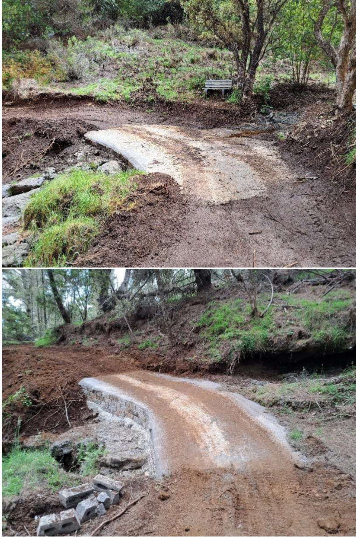
Figure 6. We repaired spillways #6 and #13 with steel-reinforced cement crossings.
