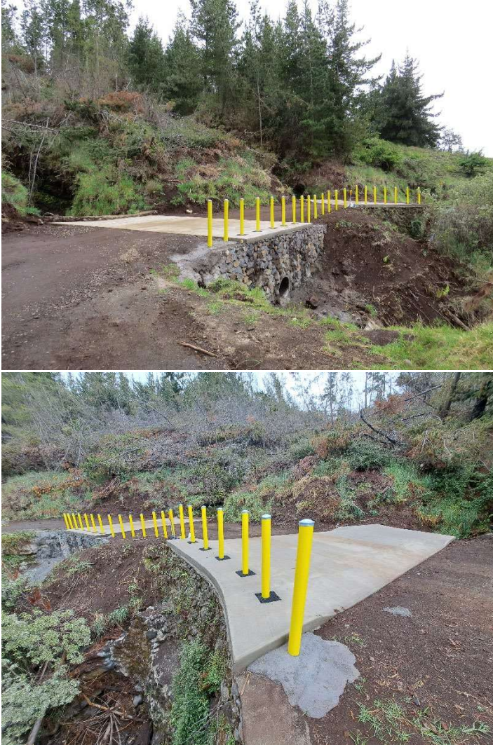
Figure 4. Newly reconstructed culverts and spillways after repairs.
