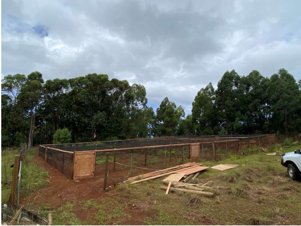
New fly pens constructed, Kauai
