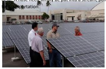
An array of photovoltaic panels provide the necessary power to run the electrolyzer and no fossil fuels are utilized anywhere in the hydrogen creation process making it a totally renewable resource.
