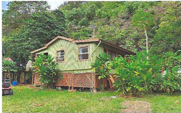
Photo 5. Property Manager's residence.
