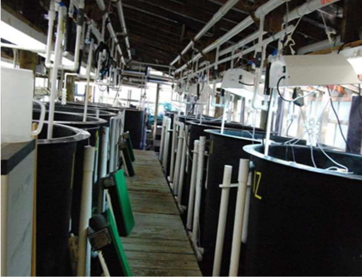
Fig. 1. Oceanic Institute’s fish and shrimp hatchery. Note the “open air” design which compromises biosecurity and environmental control.
