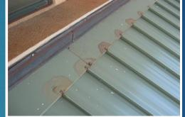
Moderate to severe corrosion of flashing.
