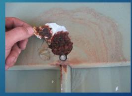
Corrosion of underlying ferrous metal.
