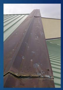
Unsecured and unsealed lap seam in expansion joint.
