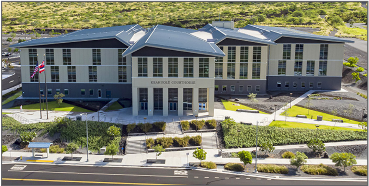
The Keahuolū Courthouse, Kona, Hawai'i island. Photo courtesy of AHL and Andrea Brizzi Photography, 2019.
