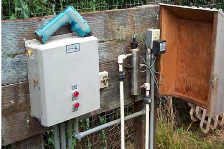
Figure 3.11 An ultraviolet disinfection system (steel cylinder to the right of the control box) used to treat sand filter effluent before landscape irrigation
