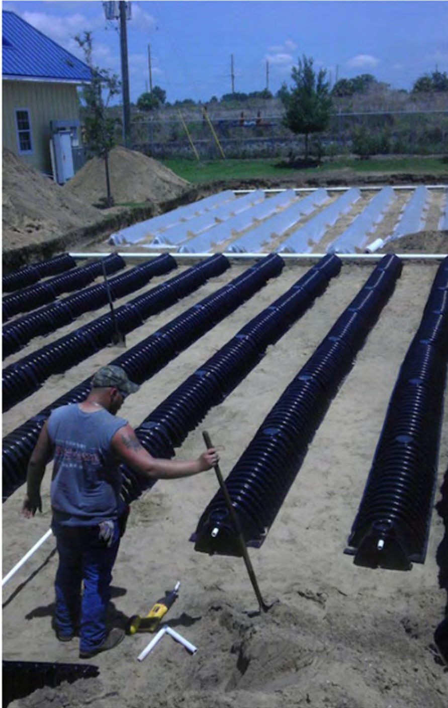
Figure 4.13 Typical Gravelless Absorption Bed Disposal System (Infiltrator.com, 2020)
