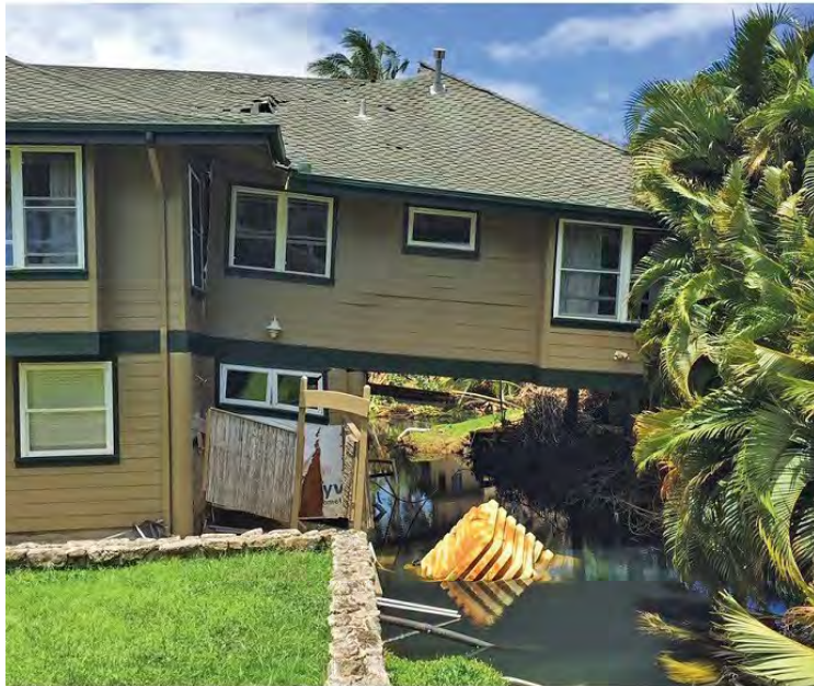
Figure 2.5 Significant Rainfall in April 2018 Caused a Septic Tank to Float in Hanalei, Kaua'i 6
