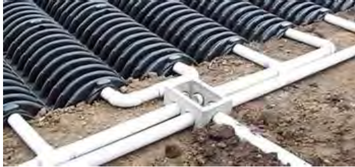
Figure 3.19 Infiltrator™ Gravelless Drainfield System (Infiltratorwater.com, 2020)
