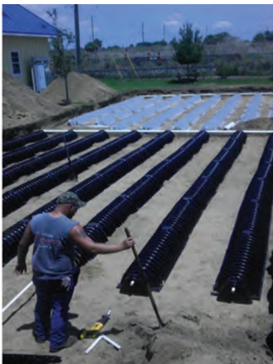
Gravelless Absorption Bed Disposal System.
