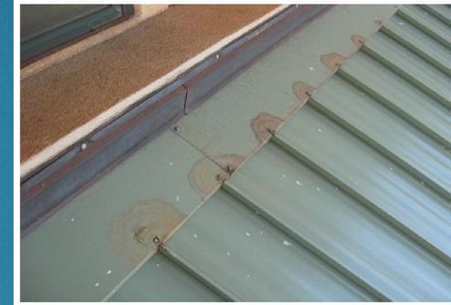
Moderate to severe corrosion of flashing.
