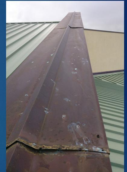
Unsecured and unsealed lap seam in expansion joint.
