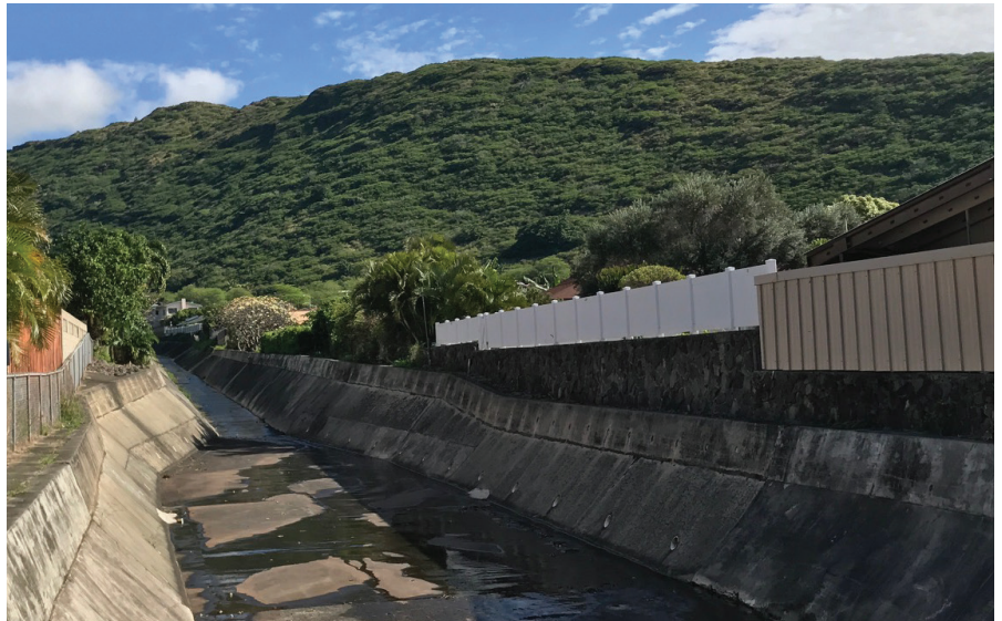
Recently cleared East Niu Stream
