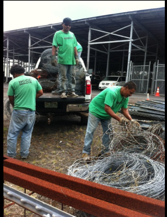
Barbed wire removal
