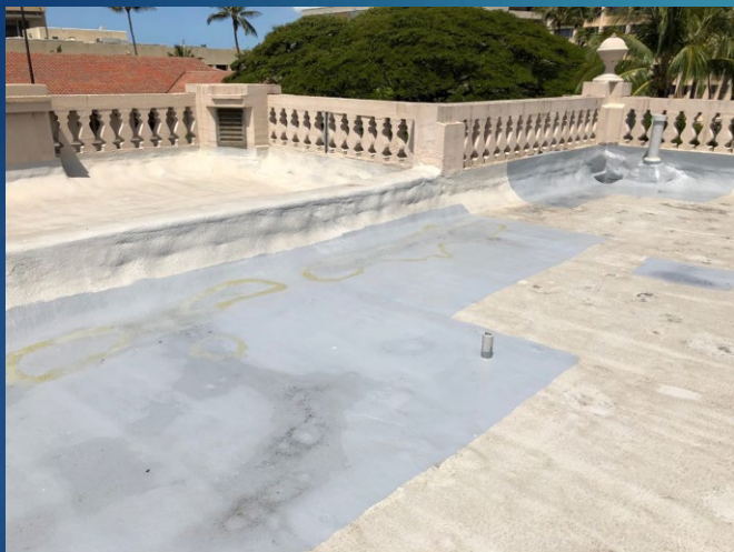
Temporary repairs along the parapet.
