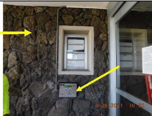
After photo of the newly installed intercom System
