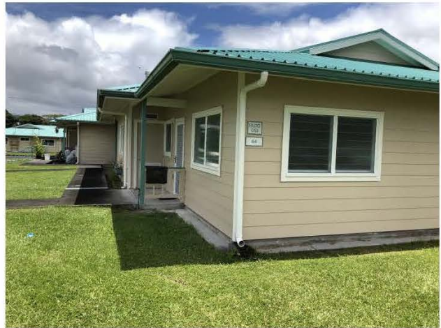
After: Building exterior was repaired, including the installation of new roof panels.
