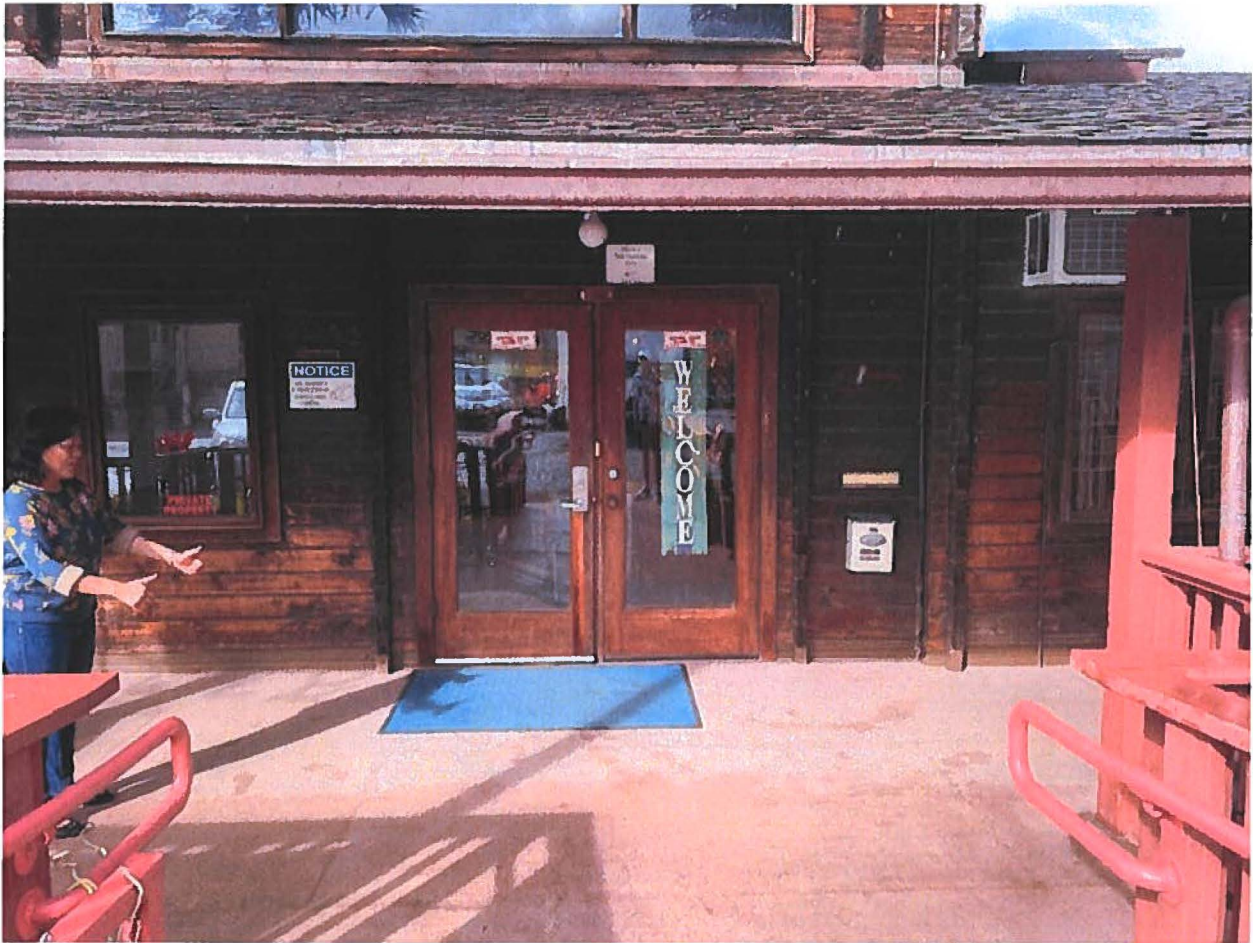
Photo 13: Front Entrance Doors
