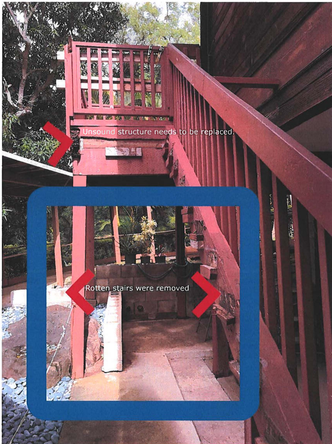
Photo 7: Lanai – Stairs to lower level were demolished for safety.
