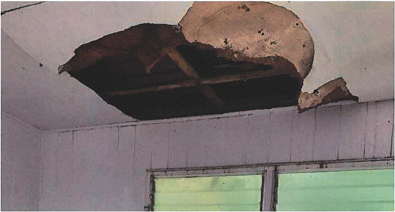
O'ahu Ranger Cottage – Ceiling in Hawai'i Nature Center Administrative Space
