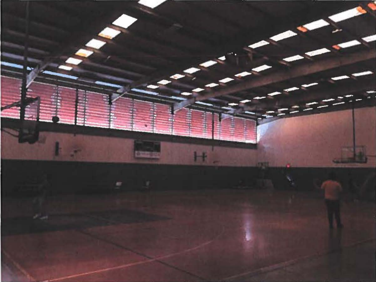
Interior photo of gym needing Renovation.
