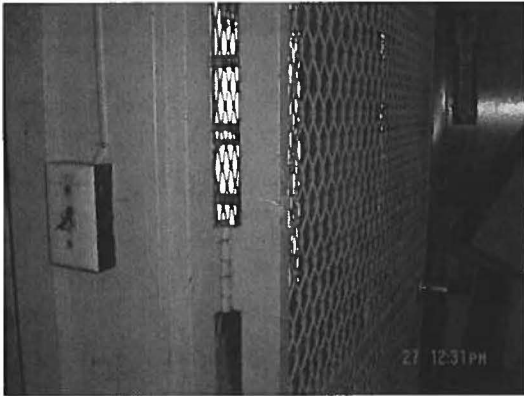
Sample no: 305-P19. Shower-Locker Room. Green metal equipment cage storage area. LBP 27,000 ppm
