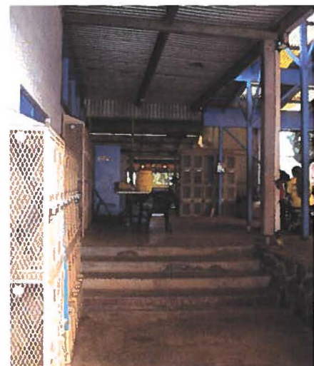
Figure 26 Classroom Chain Link Wall
