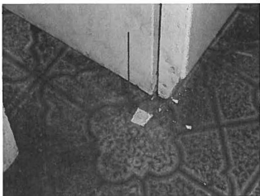
Sample no: 305-A11. Kitchen, Room 10. Burnt-orange vinyl floor tile w/ mastic.
