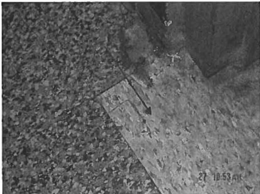
Sample no: 305-A10. Game Room. Speckled tan (patch) vinyl floor tile w/ mastic.
