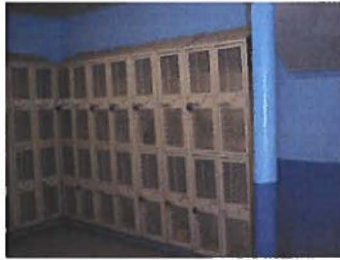
Figure 13 Existing Locker Room
