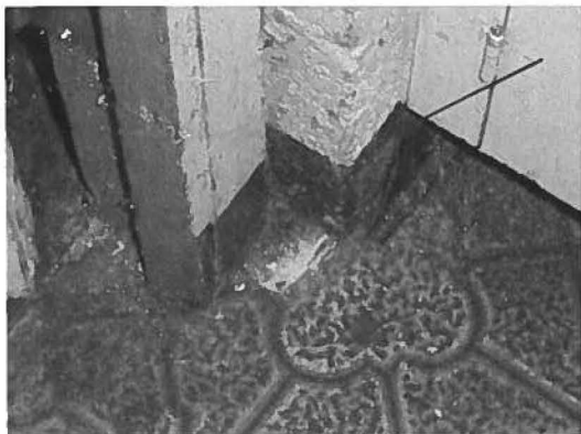
Sample no: 305-A12. Kitchen, Room 10. Brown covebase w/ mastic. ACM 35% Chrysotile (covebase)
