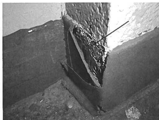
Sample no: 305-A6. Game Room-Lounge Area. Brown covebase w/ mastic (covebase is painted light blue).
