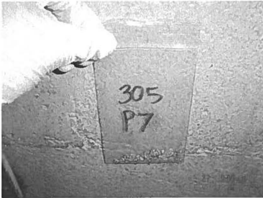
Sample no: 305-P7. Gymnasium. Blue concrete block interior walls. LCP
