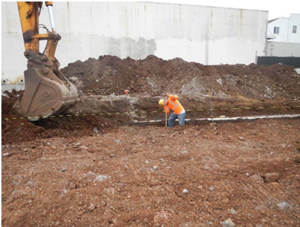
Contractor Measures the Depth of the Excavation to Ensure Enough Contaminated Soil is Removed at Lagoon Station.
