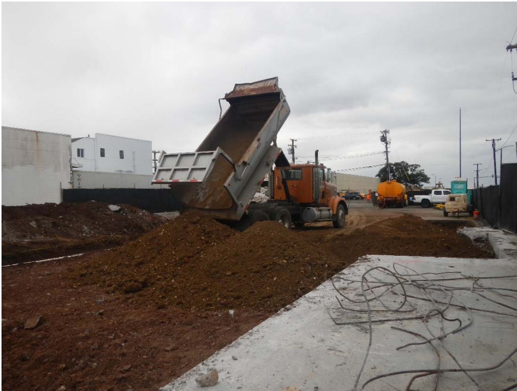
SHWB and HEER Office Oversight of Soil from Other Rail Construction Locations Used as Fill at Future Lagoon Station
