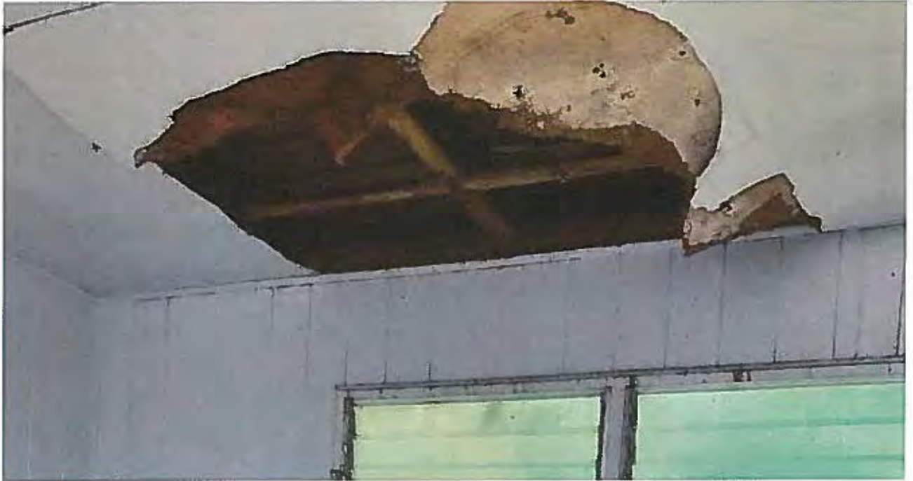
O'ahu Ranger Cottage – Ceiling in Hawai'i Nature Center Administrative Space
