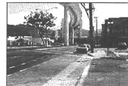
To pass above H-1 Freeway at University Avenue, the rail structure would be elevated as much as 60 feet, according to city officials.
