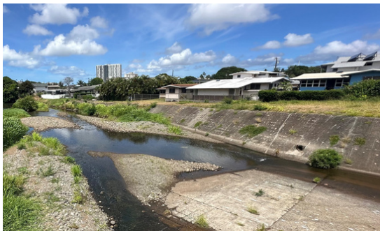
View of Halawa Stream from Salt Lake Blvd, near McDonald's
