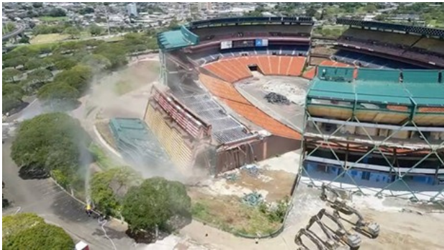
The yellow sections of the stadium is dismantled
