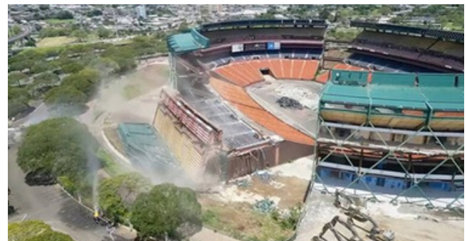
The yellow sections of the stadium is dismantled
