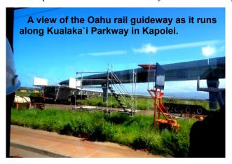
More than 5,200 massive concrete trusses – each weighing 50 tons – are being put in place atop columns for the first ten miles of the rail guideway. The tracks for rail cars sit on top of all of that.
