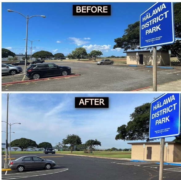
Pictured: newly paved Hālawā District Park parking lot.
