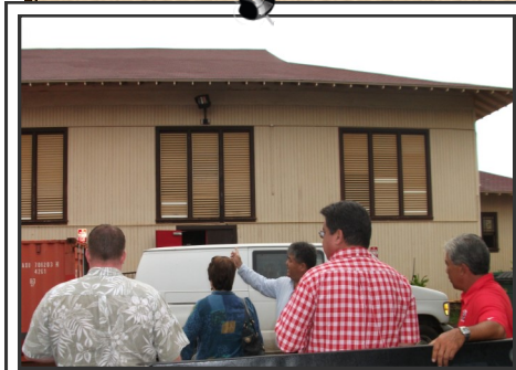
KAWAI HIGH SCHOOL GYM IMPROVEMENTS $10,936,000
