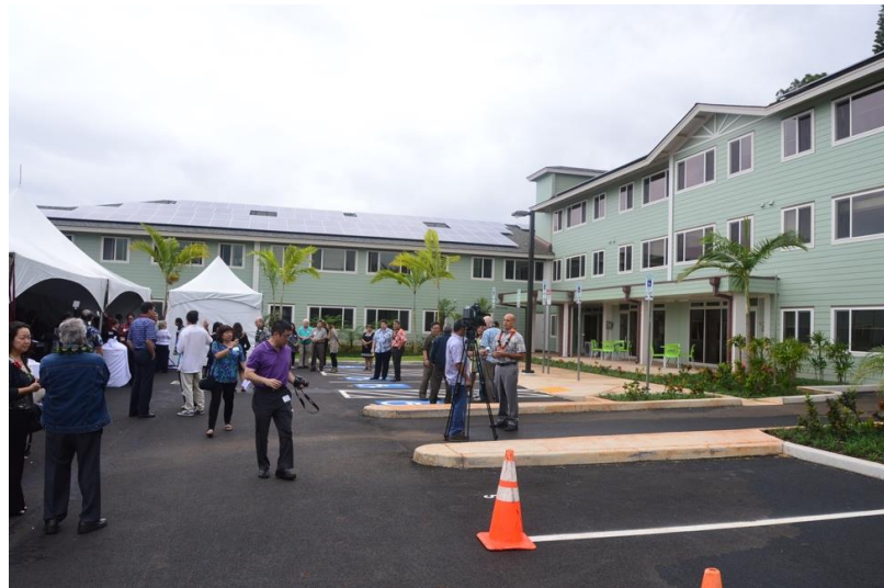
Meheula Vista Senior 301-unit master planned community for seniors located in Mililani, Oahu. Meheula Vista will provide low-income seniors an affordable permanent living option where residents can age in place.
