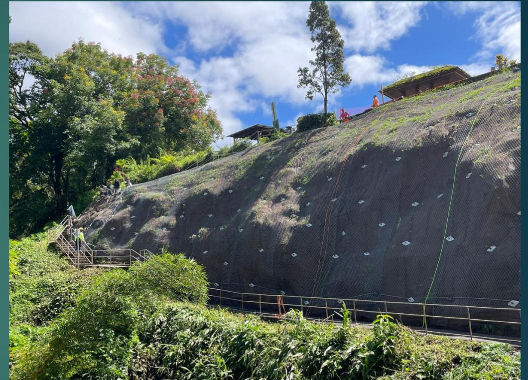
Akaka Falls Rockfall Mitigation, Hilo, Hawaii – Installation of a draped-anchored mesh system (September 2024)
