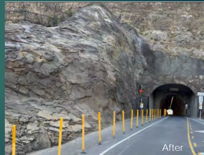
Diamond Head State Monument (DHSM) Rockfall Mitigation, Oahu – Installation of grouted anchors, structural and sculpted concrete, and tunnel entrance concrete structure. (Completed July 2025)
